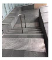
316 polished stainless steel plate complete with 316 Stainless steel carborundum infill tactiles. Tactiles come with either black or yellow carborundum inserts
